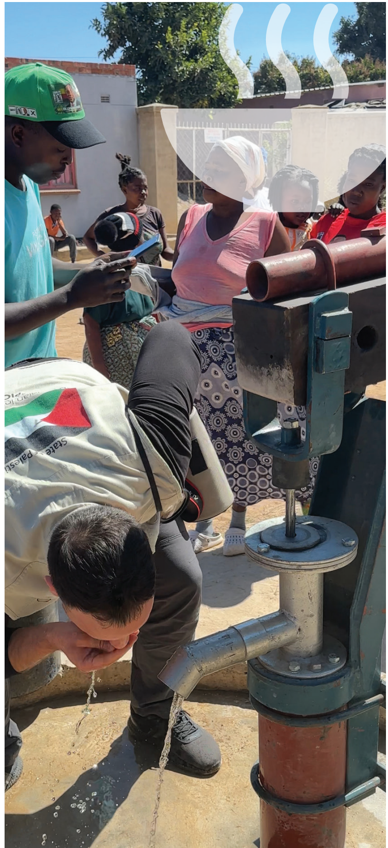
The installation of seven boreholes in Harare, Zimbabwe.
